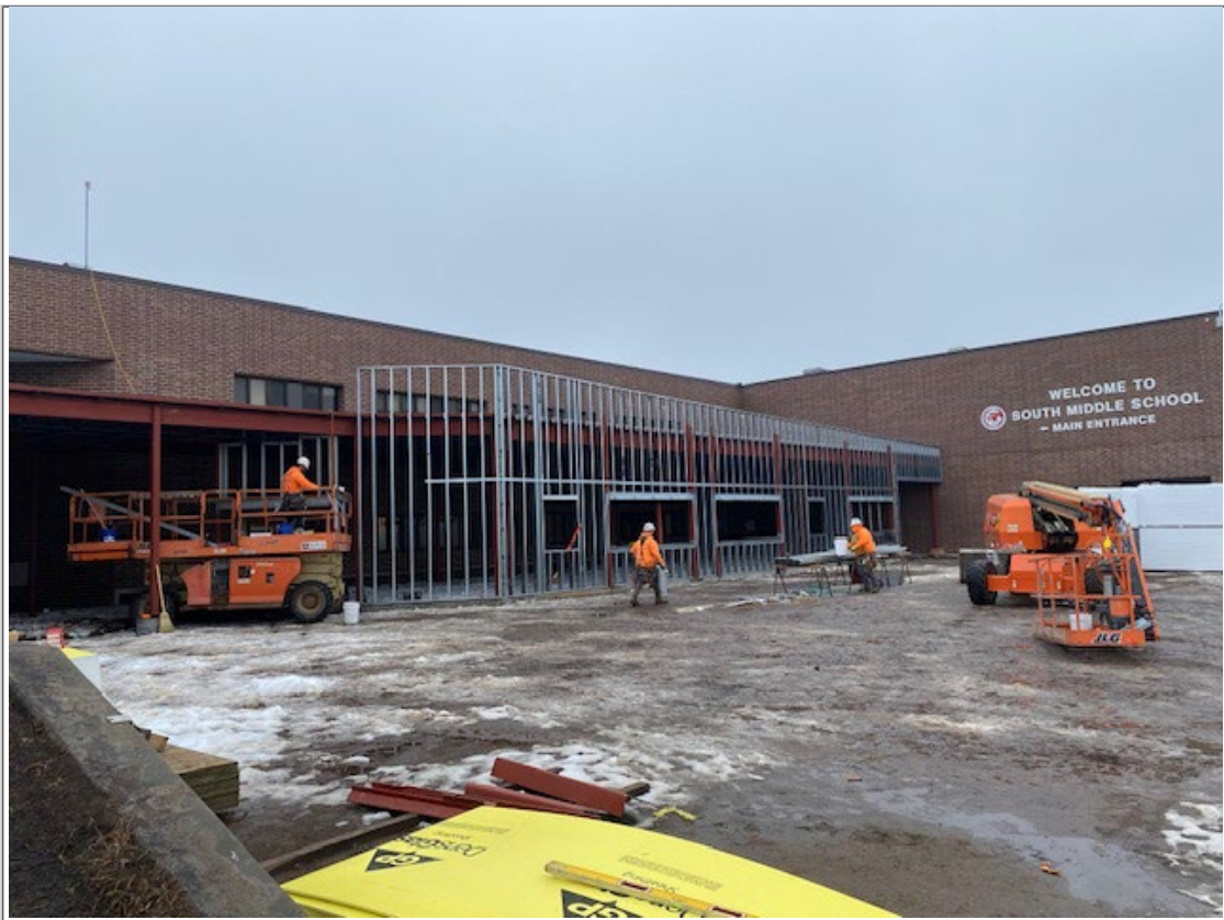
Framing front entrance
