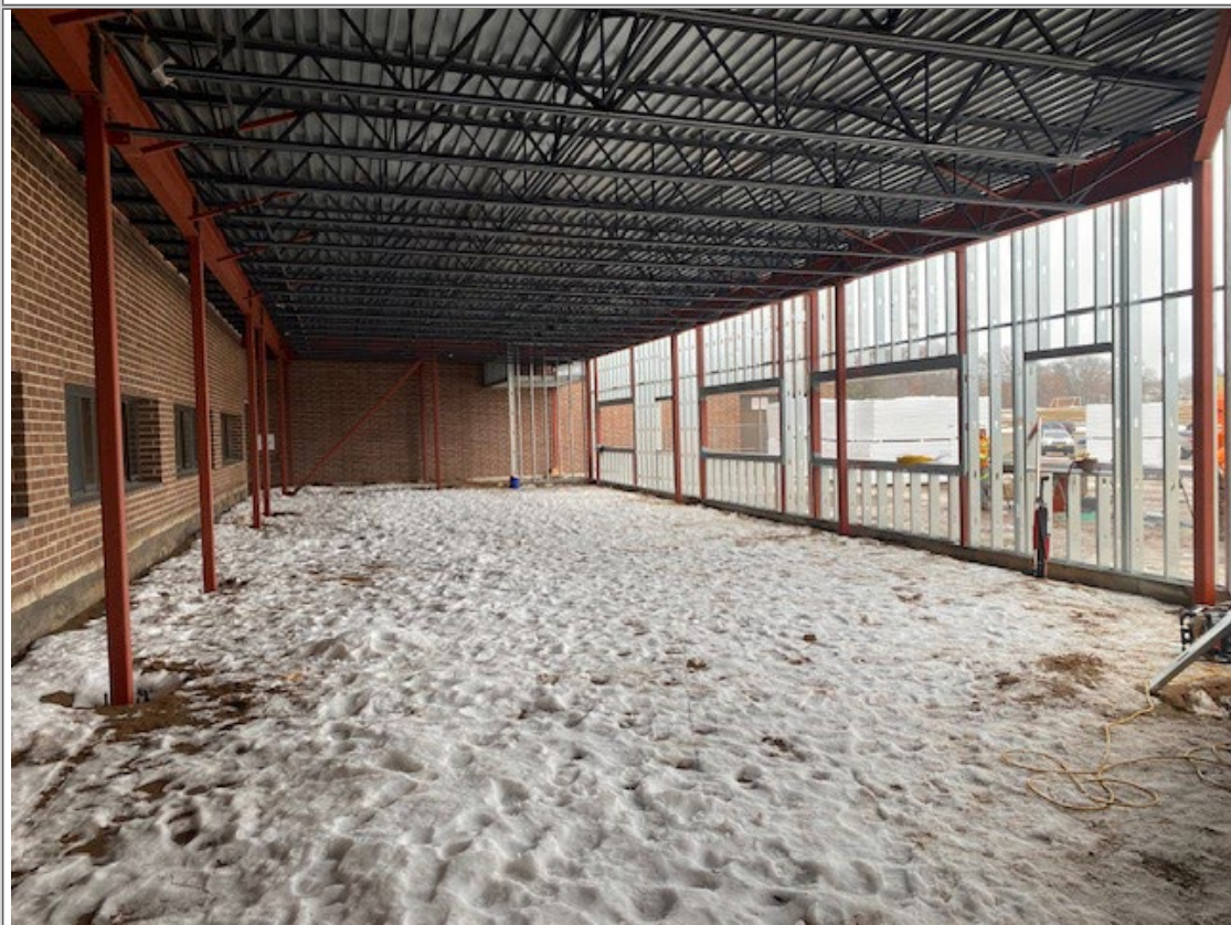
Setting Steel Area D front entrance
