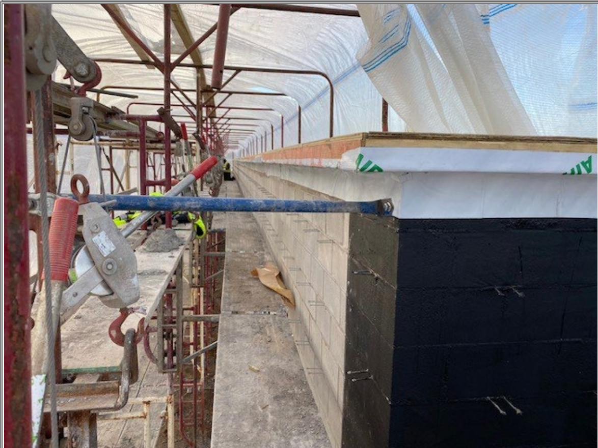
Roof cap on East wall.
