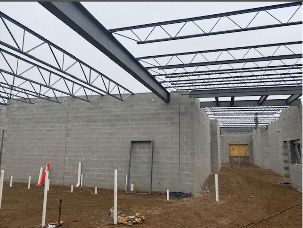
Bar joist in corridor looking North.
