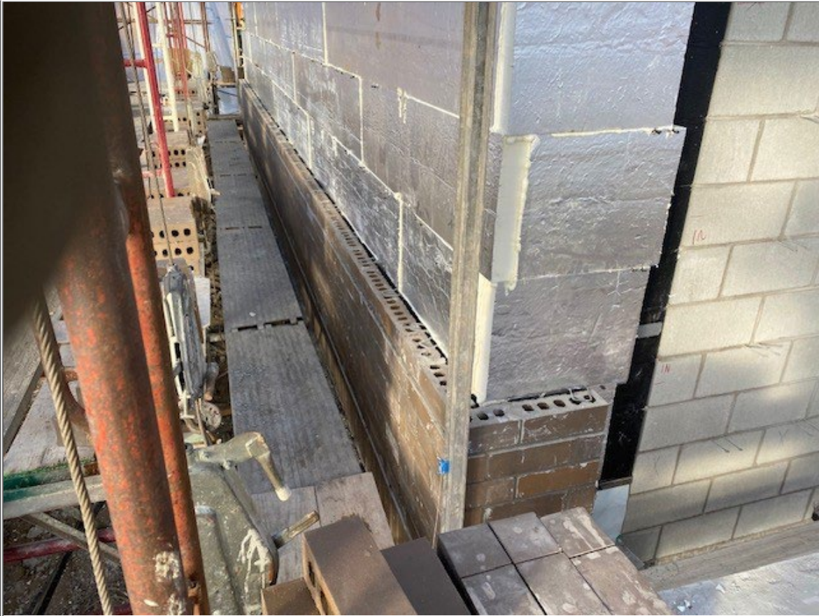
South wall brick under construction.
