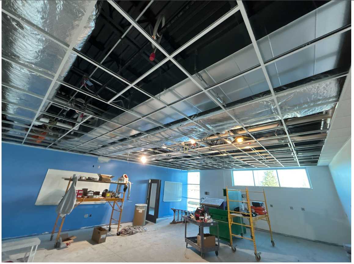
Ceiling Grid Installed
