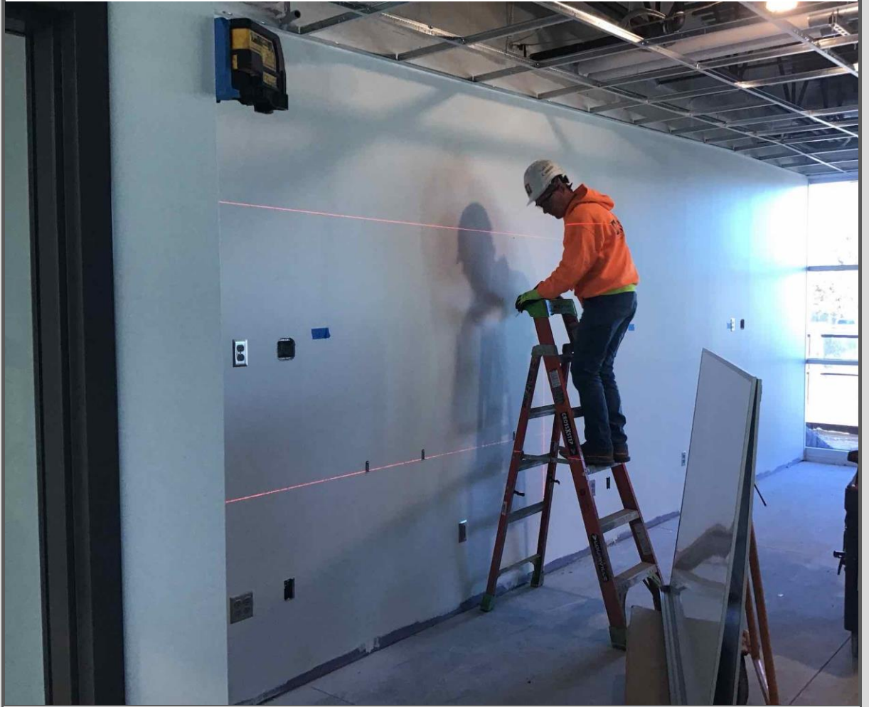
Installing Marker Boards
