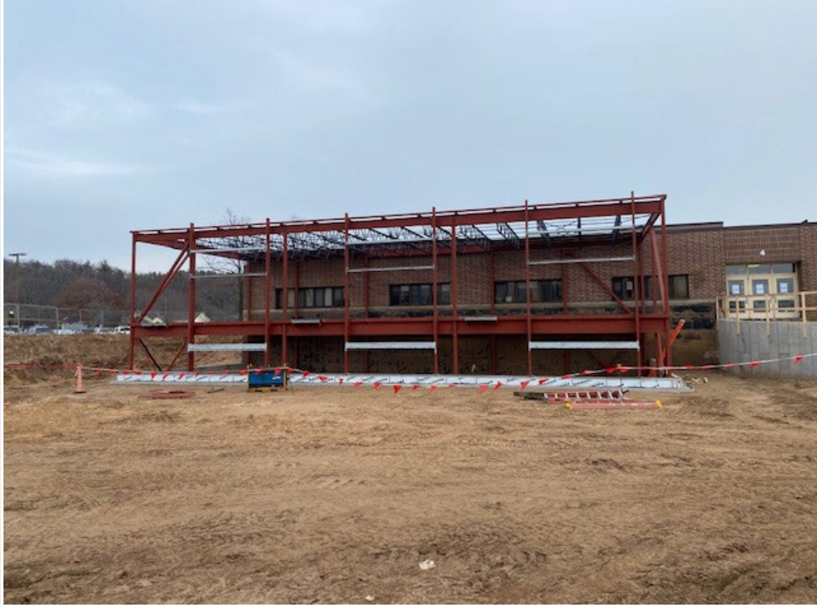
Structural steel area A
